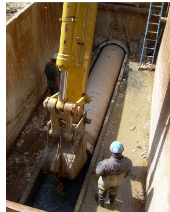
Trunk Line Rehabilitation Slip Lining
