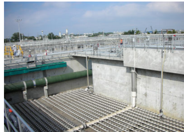
Plant Upgrades Aeration Tank
