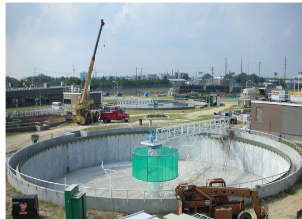
Plant Upgrades Primary Clarifier
